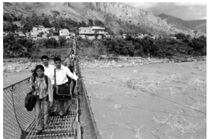
PBI volunteer Jenny Brav with Jagat Biswokarma (Dalit Human Rights Organisation), and Lal Prasad Sharma (Federation of Nepalese Journalists) on a river crossing in Myagdi District, Eastern Nepal. Jenny, together with Andrew Miller, undertook the trip to understand the pressures faced by human rights groups including Dalit, ethnic groups, and women's rights activists, and to get feedback on the protection workshops and the role that PBI could play.
